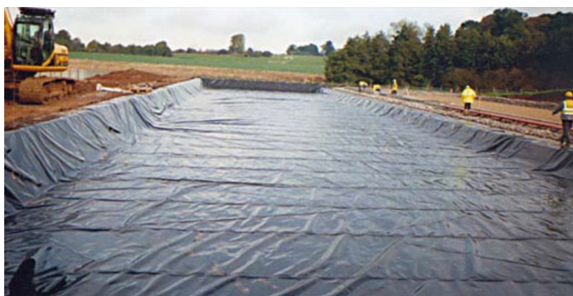
Figure 3.32 A lake liner: polyester multi-split fibre gauze/scrim sandwiched between two LDPE films. (photo: Keytec Environmental Ltd)
